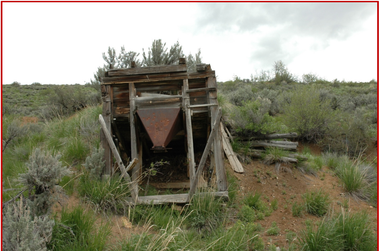
Figure 57. Ore loading bin (front view) in lower Coleman Canyon (taken June 9, 2010).
